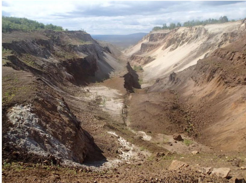
Figure 7.23: Strong Sanding in the Illinois Creek Central Pit
